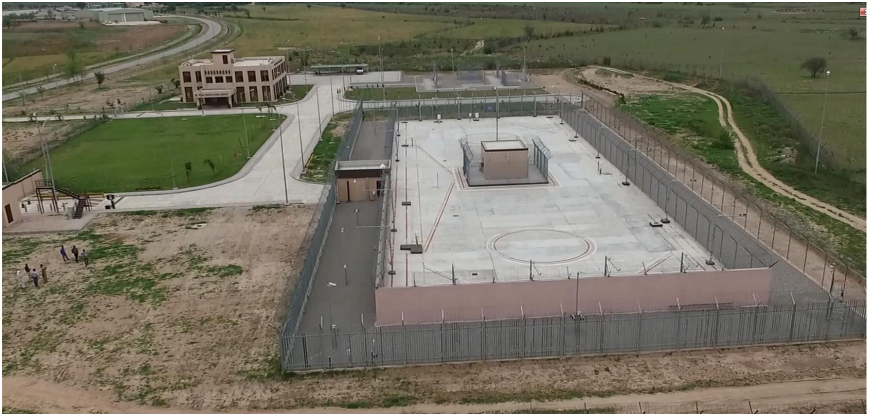
Physical Protection Exterior Lab
